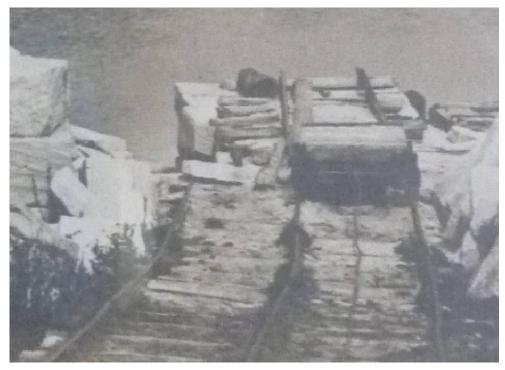
**Figure 3.14** Detail of photo of quarry wharf held by Mosman Library. Note the wharf appears to end abruptly to the left (north) of the tracks and the steep slope of the tracks.
